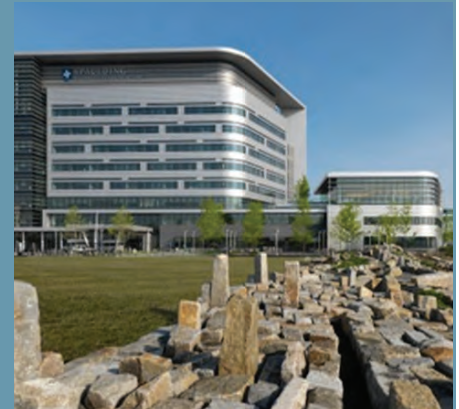
Figure 11: Spaulding Rehabilitation Hospital, completed in 2013 on the Boston waterfront, includes such resilience features as an elevated first floor and roof-mounted electromechanical infrastructure.
