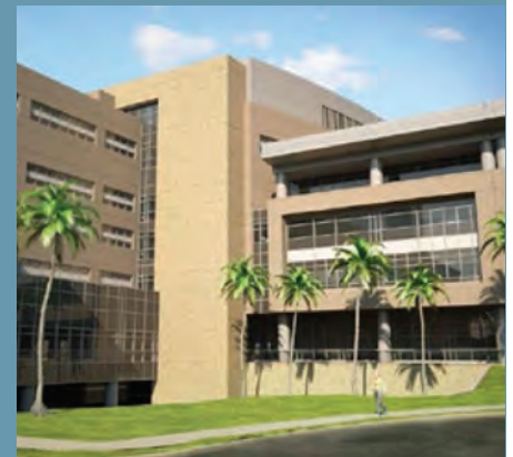
Figure 2: The new clinical services building at UTMB consolidates departments formerly housed in hospital buildings at or below grade
