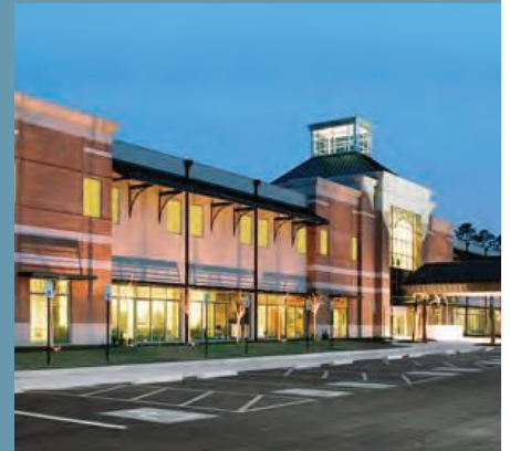
Figure 15: Louisiana Heart Hospital, designed to withstand high winds, successfully operated through Hurricane Katrina
