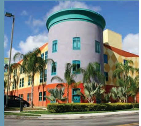
Figure 1: Miami Children's Hospital retrofitted its façade to withstand hurricane force winds.
