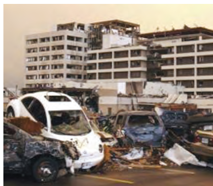
Figure 22: Debris outside the Joplin Hospital Emergency Department, following the EF-5 tornado, complicated evacuation procedures.
