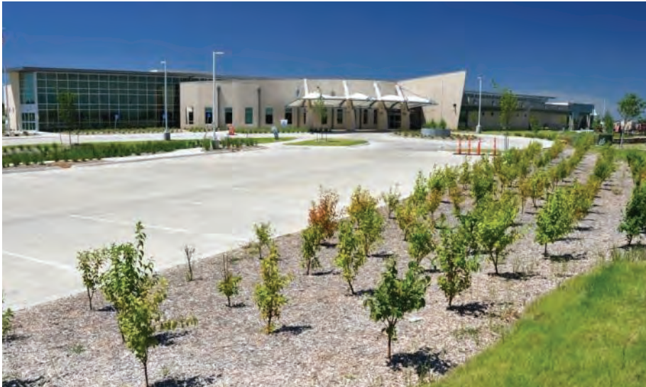
Figure 25: These bioswales at Kiowa County Memorial Hospital filter stormwater and support the Ogalalla Aquifer recharge. Rooftop rainwater is collected for irrigation and toilet flushing.
