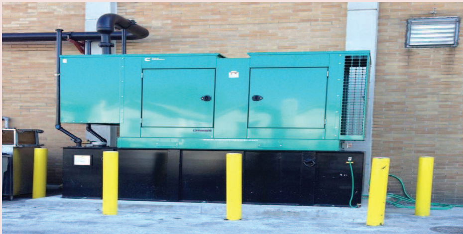
At Shore View Nursing Home in Brighton Beach, an emergency generator was moved from the basement and elevated on a raised platform.
