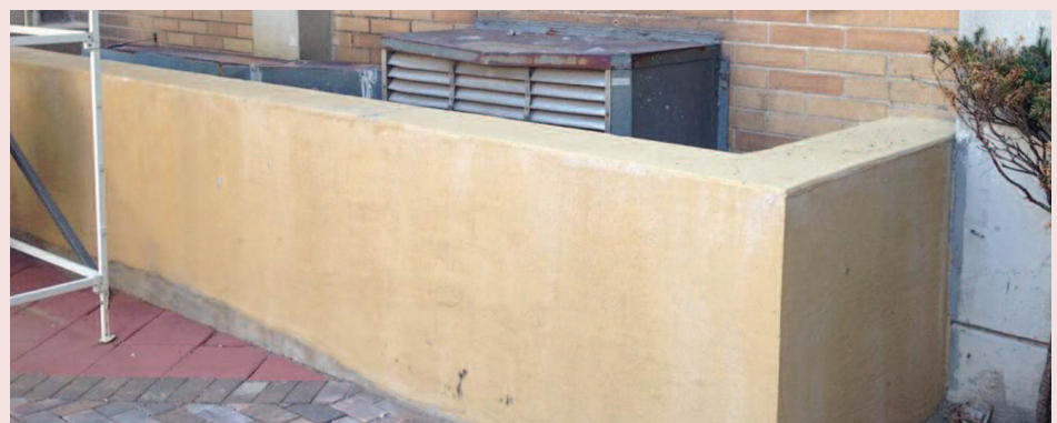
At Shore View Nursing Home in Brighton Beach, a cement wall protects vents for boilers and chillers from over 5 feet of storm surge.
